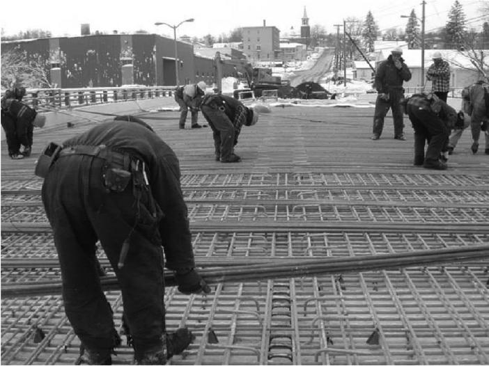
Figure 1.6 GFRP reinforced-concrete bridge deck (Cookshire-Eaton, Quebec, Canada).
