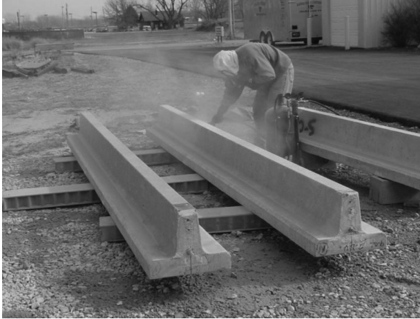
FIGURE 8.4 Surface preparations by sandblasting.
