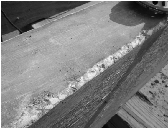
FIGURE 8.5 Rounded beam corners by grinding.
